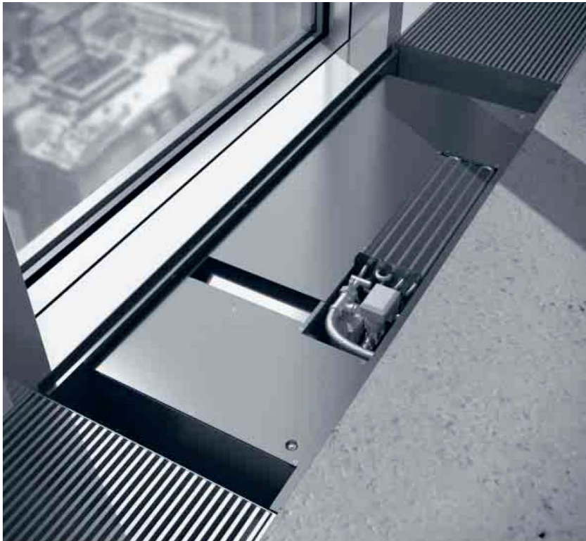
LHRV fancoil integrated in floor or ceiling: with central heating & cooling + local ventilation ('Fassaden-belüftung', Schüco).
