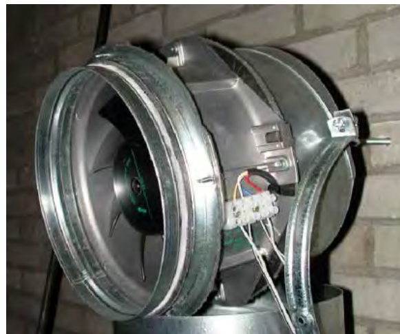
Figure 5- 9: Example of axial fan for continuous fan-assisted residential stack ventilation. SFP is 0,04 kW/(m^3/s) at nominal flow 10 Pa & 56 \ell/s with 2 W^5 [26 ]. [Source: TNO] EC-motor fan with system efficiency 28%.
